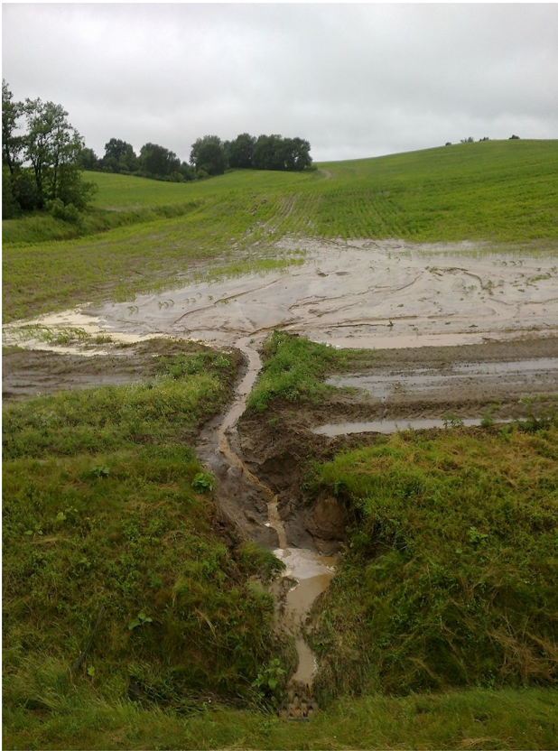
Fig. 4 Effects of soil erosion in the study area after intensive rainfall. Silt fine particles are visible as a wide yellowish-brown “plate” at the toe slope section and small erosion channels caused by concentrated runoff
